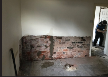
Photo 2 Internal wall repairs
